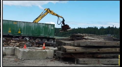
Pulled creosote pilings being processed for offsite disposal.
