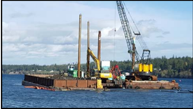
Dredging operation in SMA-1.
