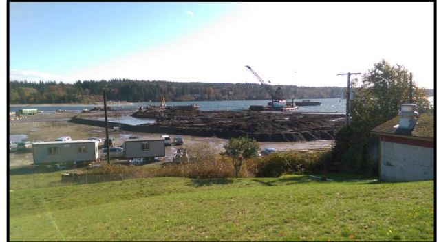
View of the containment berms for dredged sediments.
