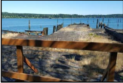
Before: The Former Log Transfer Facility
