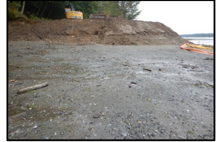
After: Pile pulling & pier demolition complete at Former Log Transfer Facility
