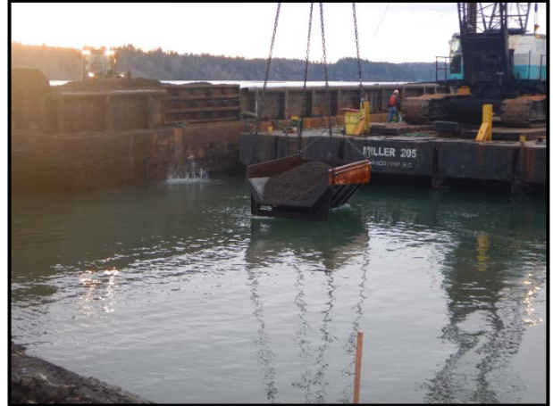
Placement of 3" minus backfill.
