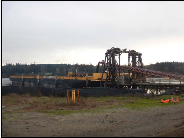
Capping materials being loaded onto a barge.
