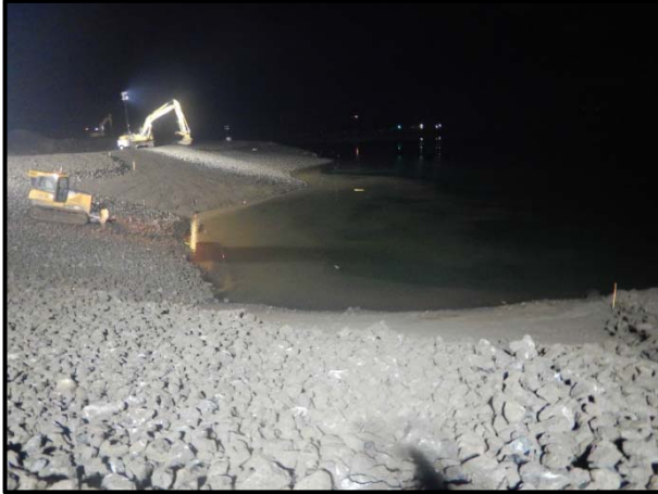
Pier 4 capping area, work being done during night time low tides.
