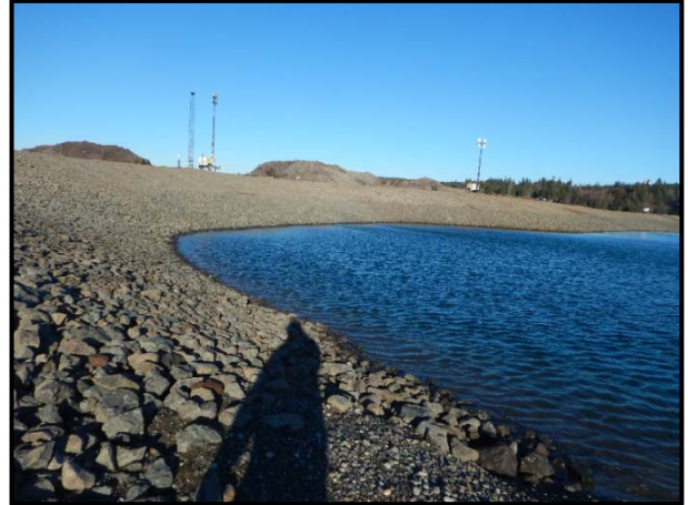
Completed Pier 4 cap.
