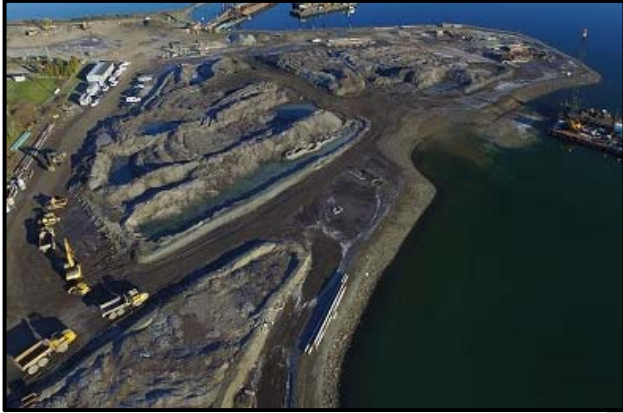
Dredged sediment stockpiles on Mill Site.
