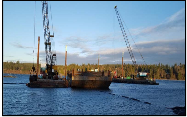
Capping operations in SMA-1.
