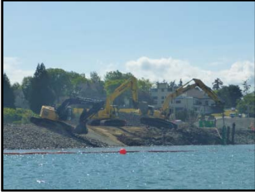
Pile removal, bank excavation and capping
