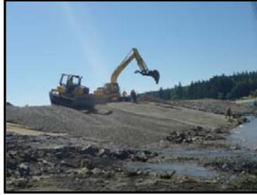
Clean capping material being placed after bank excavation completed
