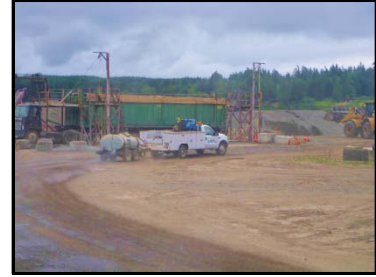
A water truck keeping the dust down during construction
