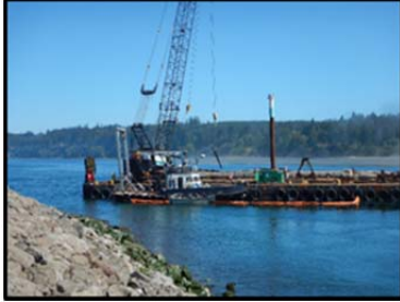
Diver assisted pile pulling
