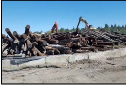
Creosoted piles ready for disposal
