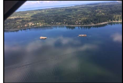
Placing clean cap in central bay
