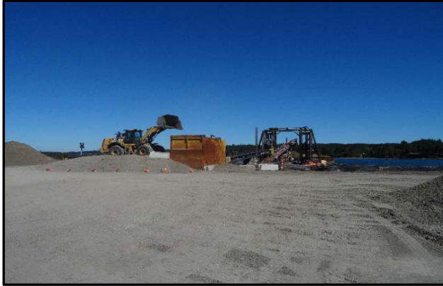
Clean capping material (sand) being put onto a conveyor for loading onto a barge.
