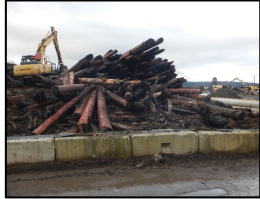
Pile processing area.
