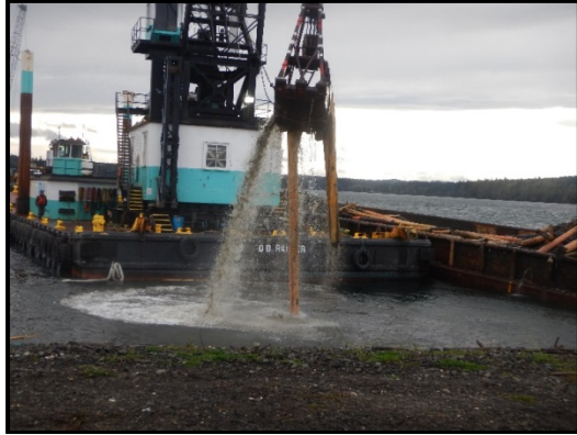
Pilings being removed during SMA-2 dredging.
