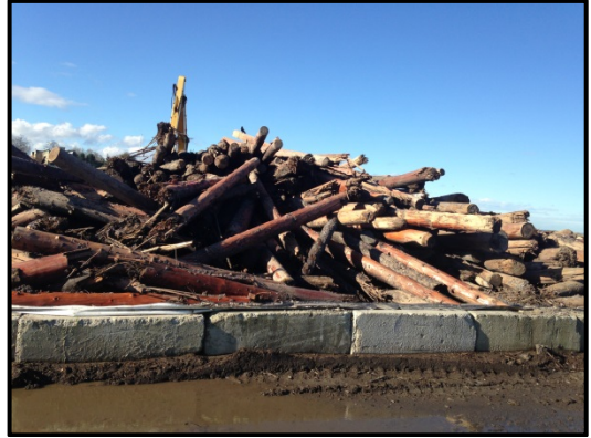
Barkies and creosote pilings pulled from the bay.
