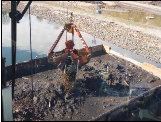
Dredged wood waste being loaded onto a barge.
