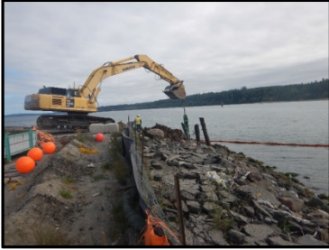
Before: Removal of intertidal piles and asphalt from Eastern Wharf.
