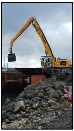
Subtidal dredge spoils being offloaded from a barge.
