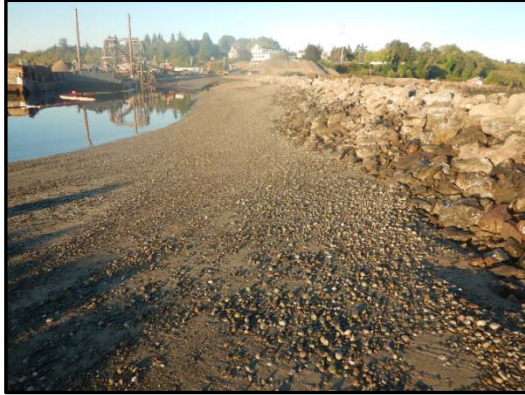
Completed intertidal cap along the jetty, north of the mill site
