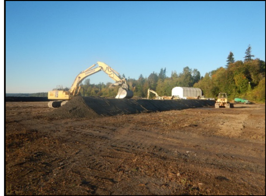
Building containment berms
